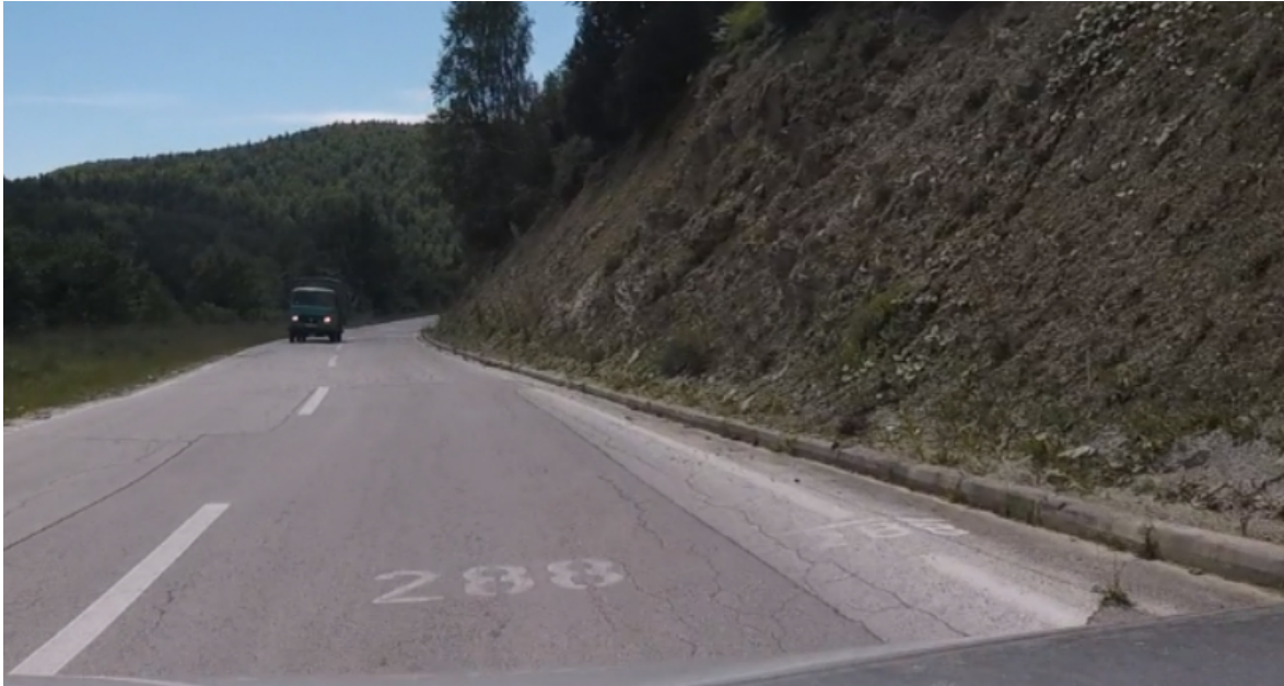
Picture 4. End of the section-border between Ivanjica and Sjenica municipalities (approx. chainage km 288+251)
