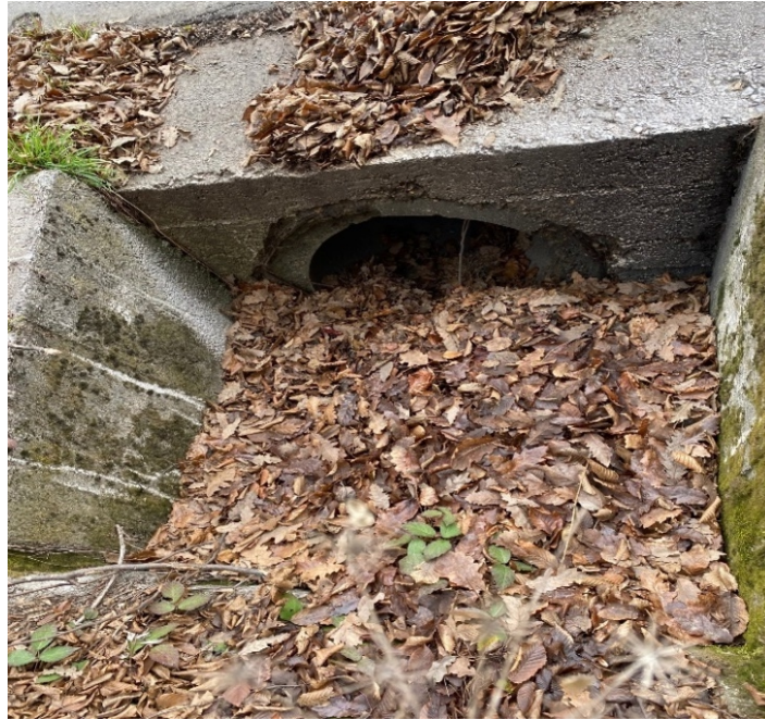
Picture 6. Pipe culvert
